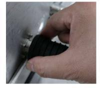
Keep twisting and pushing up until the boot is fully extended to reach the connector base of the RRU and the connector is covered 360degrees uniformly.
