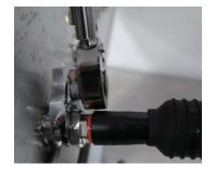
Push from the back of the boot up towards the RRU connector from one side of the boot. Opposite side is where the power and FO cables are located.
