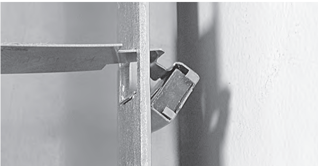
4.1 Fix the first cage nuts into the rack profile using the CAGE-NUT-TOOL.
