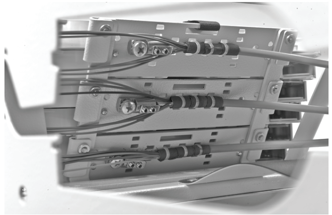
5.1.13 Fasten the strength member connector. Avoid unnecessary crossing of strength member and loose tube. Secure the flex tube using three tie wrap over the foam as shown on the pictures.
