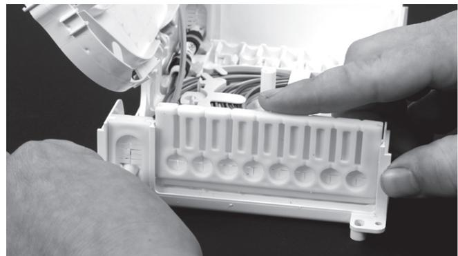
6.3 Install the seals of the box for the main as for the drop cables.
