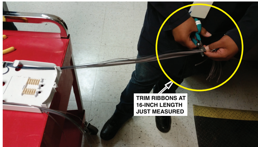
Figure 7. Trimming 1A and 1B Ribbons at 16-Inch Length
