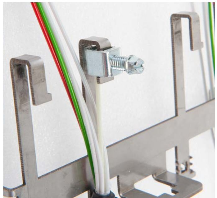
6.1.5 Secure the strength member with the metal lug.
