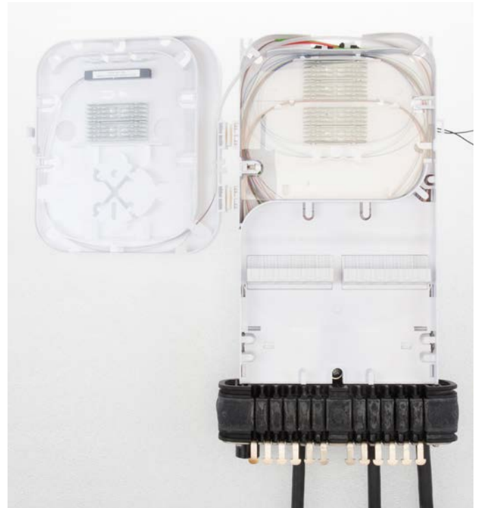
11.5 Output fibers can now be spliced to the drops.
