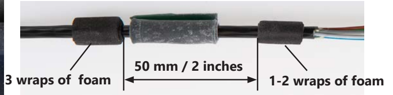
7.1.1 Apply foam tape and 50 mm gel strip.
