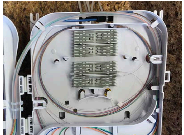
12.3 Make splices and store properly.
