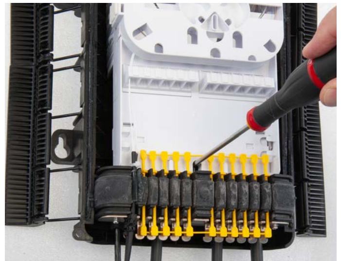
13.2 Slide organizer under the 2 top screws. Tighten 2 top and 1 bottom screw.
