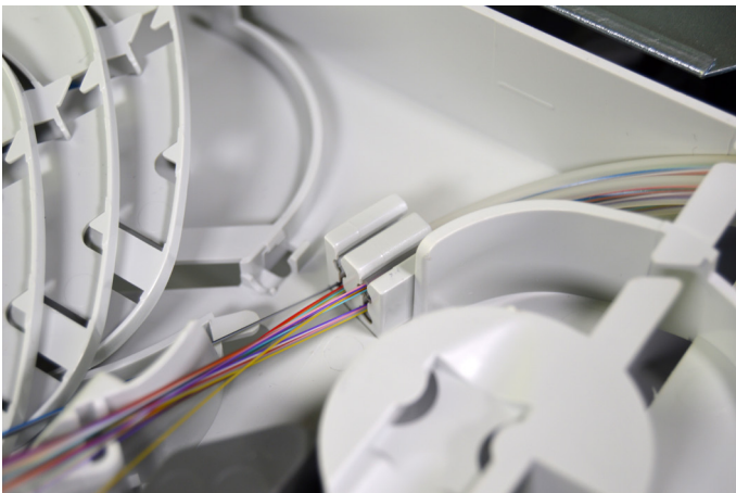
6.1.10. Push and click the tube holder into the tray. Route the transportation tubes into the FACT element.
