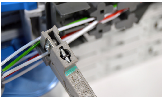
6.1.2. Strip the loose tubes at the marked point and clean the fibers.
