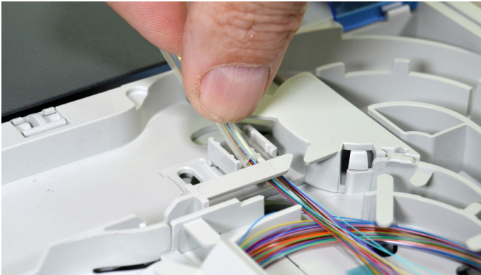
7.2.5. Place the additional tube, if needed.
